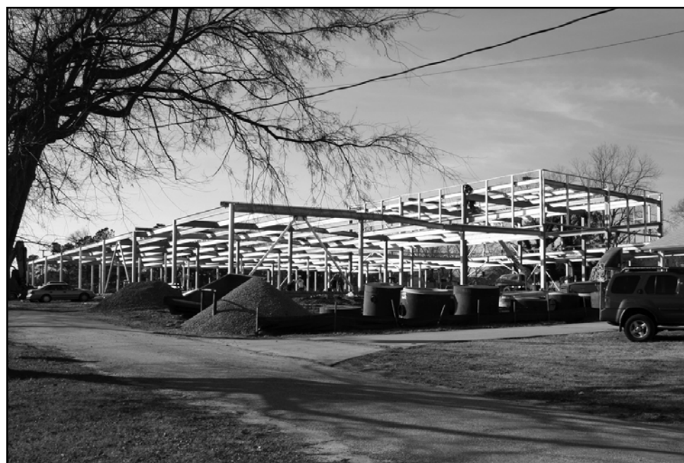
Steel framing for VIMS' new Seawater Laboratory is now in place.
