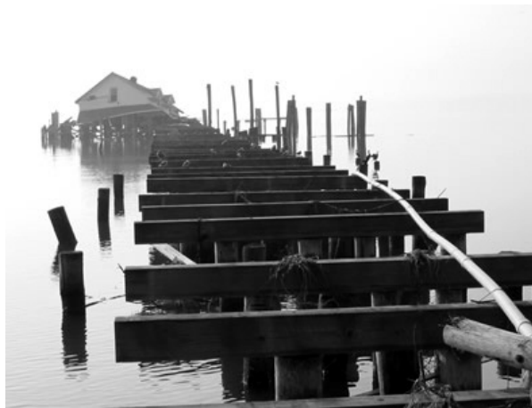
Ferry Pier and Ferry House after storm.
