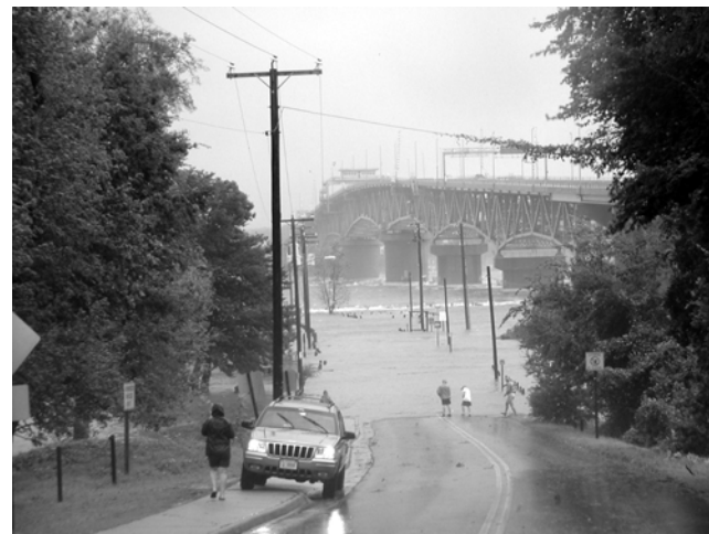
York River storm tide under Coleman Bridge.
