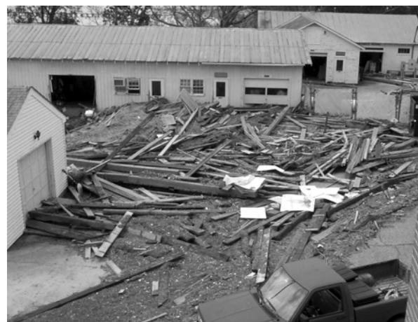
Another view of the debris in maintenance area.
