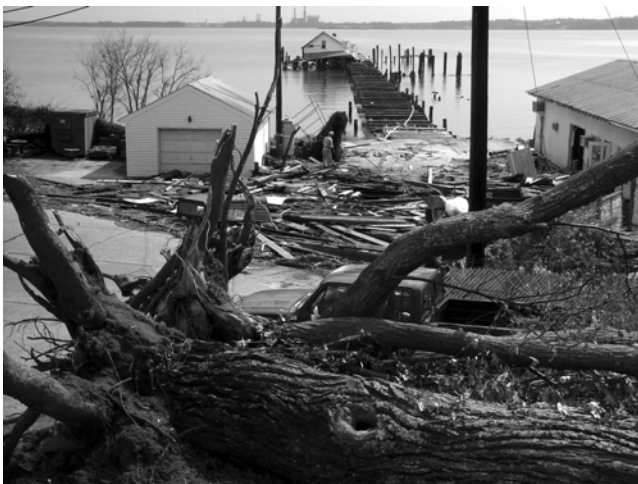
Debris and damage in maintenance area.
