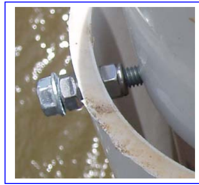
Figure 5.18 Close-Up view of a bolt-double nut
