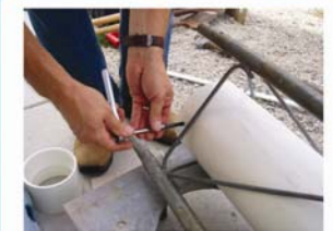
Figure 5.27 Threading top holes.
