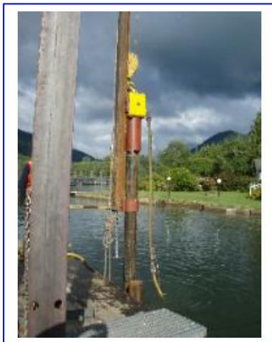
Figure 5.4 Drop hammer (Source: Whatcom Waterfront Construction)
