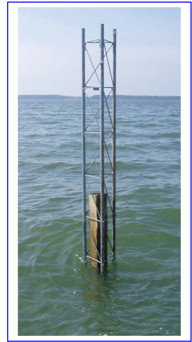
Figure 5.10 Pile station waiting for the guard-pipe to be placed.
