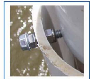
Figure 5.28 Hex head bolts with two lock nuts.
