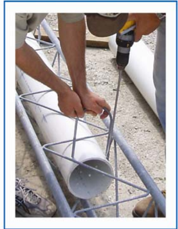
Figure 5.29 Drilling holes to place U-bolts.
