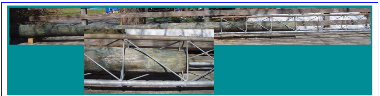
Figure 5.7 View of pile with the antenna tower mounted on land
