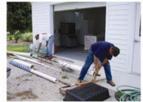
Figure 5.26 Inserting 6 foot long 6 in PVC pipe into the antenna tower.
