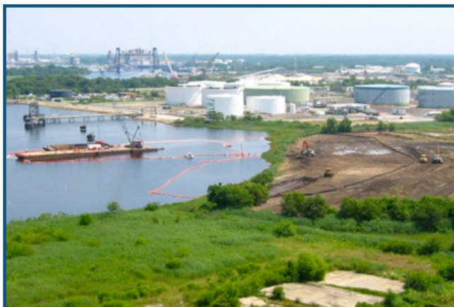
Money Point: The Money Point site during dredging of PAH-contaminated sediments. The orange boom contains the released sediment. The VIMS scientists operated the biosensor from the small boat near the boom. Photo courtesy of Joe Rieger, Elizabeth River Project.
