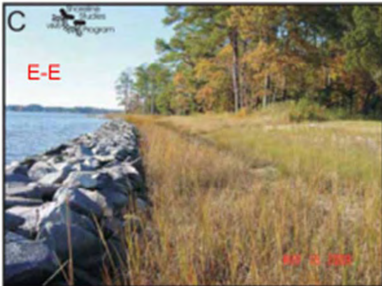
Sill system at Poplar Grove on the East River in Mathews County, Virginia six years after completion. A) The sill and marsh fringe provide a wide buffer between the water and the upland. B) The wide gap in the sill provides a pocket beach access area along the shoreline. C) The project zones are clearly visible: stone sill, S. alterniflora , S. patens , and upland/wooded. D) The old mill sits close to the shoreline. In this area, a revetment was chosen to protect the shoreline. Hardaway, Jr. C.S., D.A. Milligan and K. Duhring, 2010. Living Shoreline Design Guidelines for Shore Protection in Virginia's Estuarine Environments . Special Report in Applied Marine Science and Ocean Engineering #421. Virginia Institute of Marine Science, College of William and Mary, Gloucester Point, Va. https://publish.wm.edu/reports/559/
